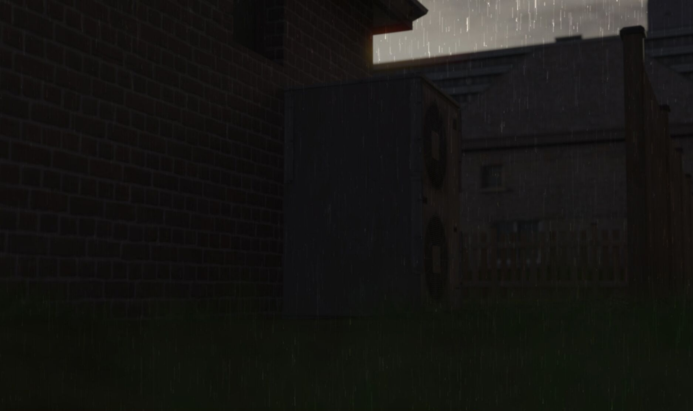
...THE OUTDOOR CENTRAL AIR CONDITIONING UNIT ON THE SIDE YARD, THE SIZE OF A LARGE CABINET, WAS LIFTED UP FROM UNDERNEATH...
